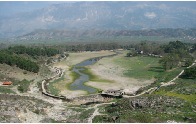
Fig. 10: Intermittent spring of Viroi, Q_{max} > 50 \text{ m}^3/\text{s} , near Gjirokaster City in southern Albania. A pumping station of 2 \text{ m}^3/\text{s} capacity is situated near the siphon; the water is used for irrigation.
