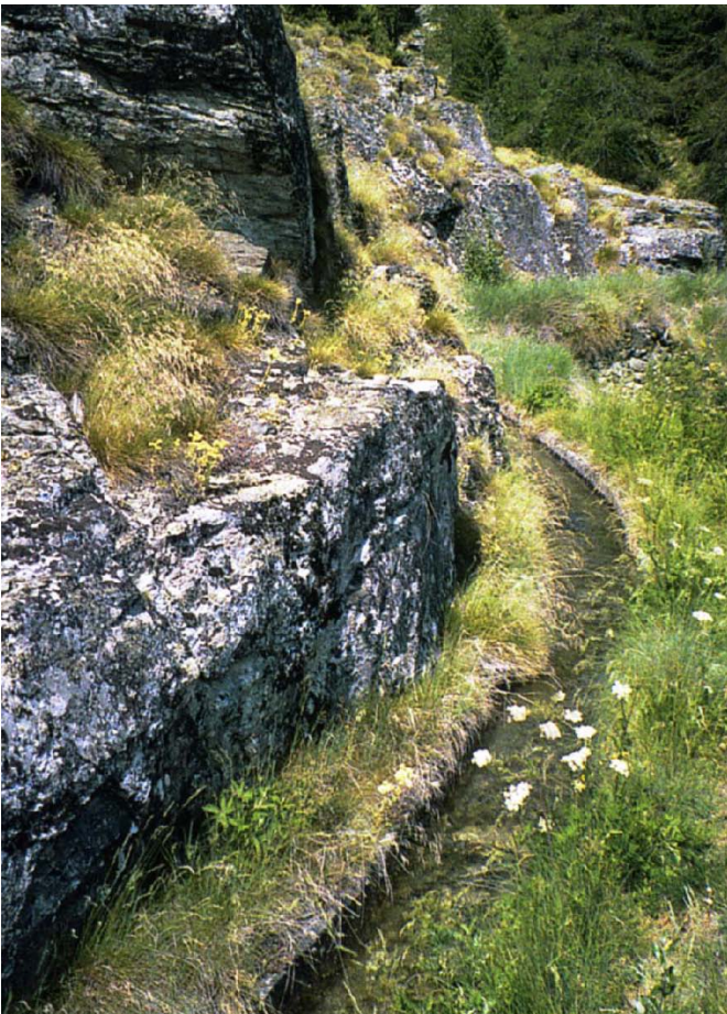
Fig. 4: Ru Vernier, irrigation canal (Quart).
