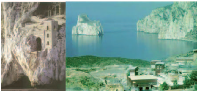
Fig. 3: On the left - The Porto Flavia mooring: the mined mineral was brought to the surface through a series of shafts tunnelling the mountain and was loaded directly onto large-tonnage ships. On the right: the Masua mining plant.
